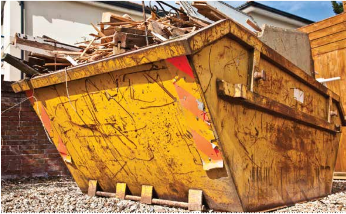
Figure 4.3. Construction Activities can Produce Significant Waste
